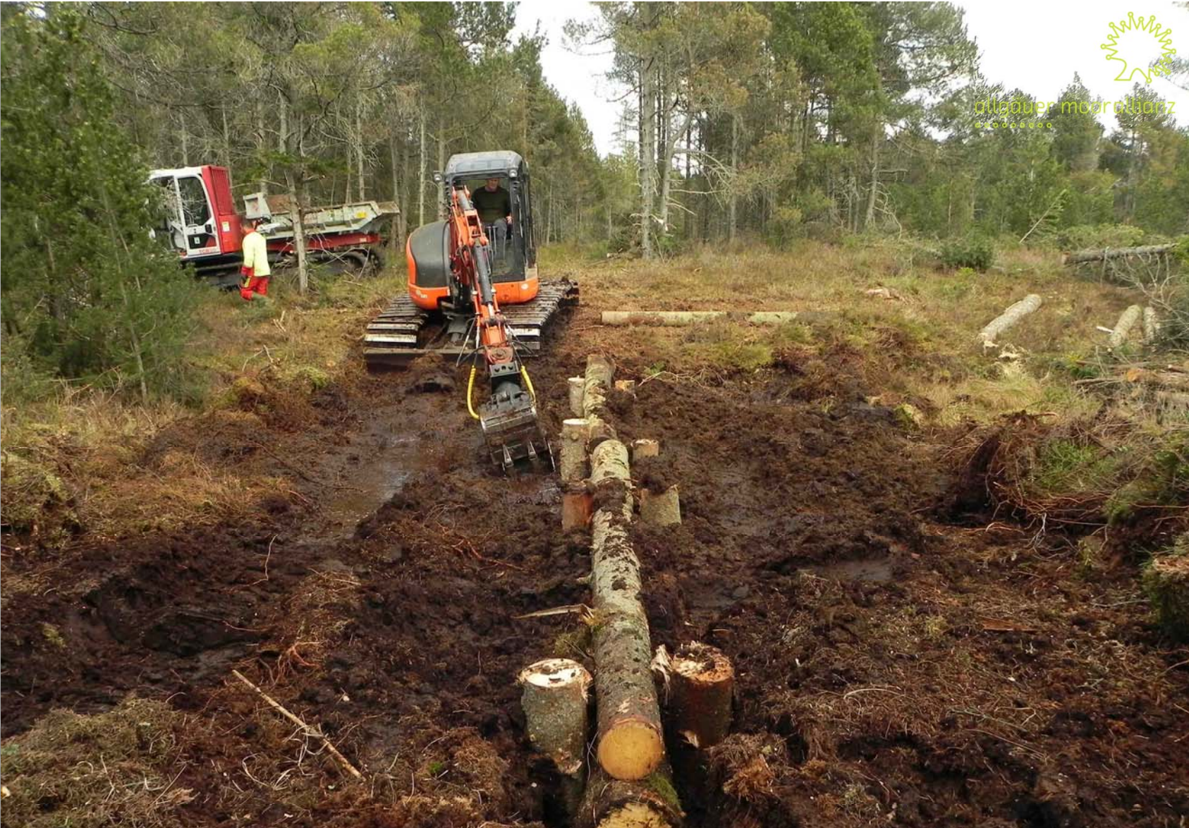
Large peat dams with log reinforcement (April/May/October 2021)
