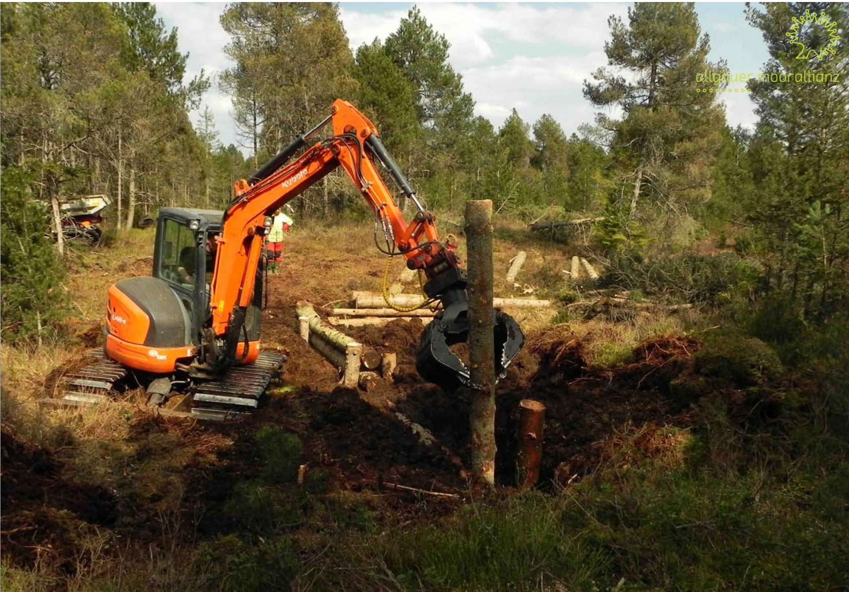
Large peat dams with log reinforcement (April/May/October 2021)
