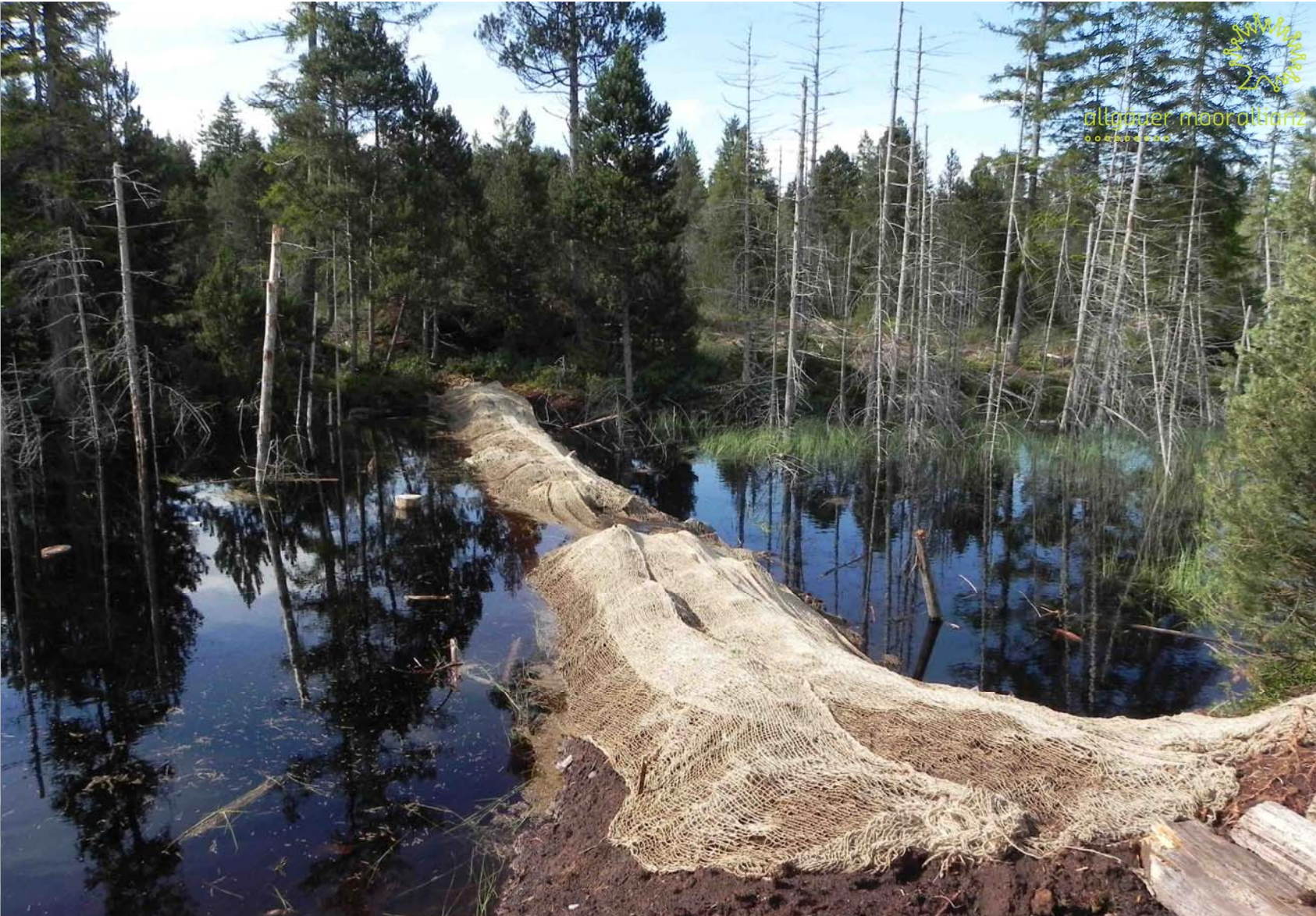
Large west-east peat mine: technical dams with steel sheet piling (July 2021)
